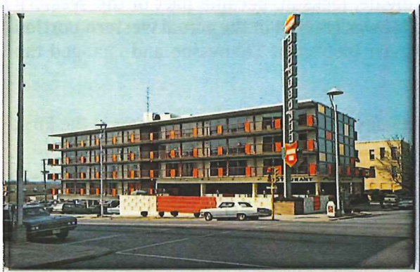
The United States Courthouse is located at the site formerly known as the Downtowner Motor Inn, Jackson, Tennessee
