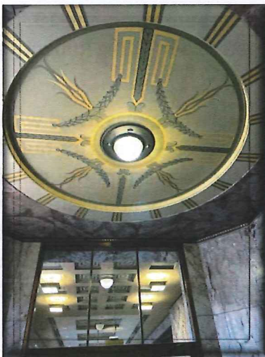
Ceiling in the alcove on the first floor
