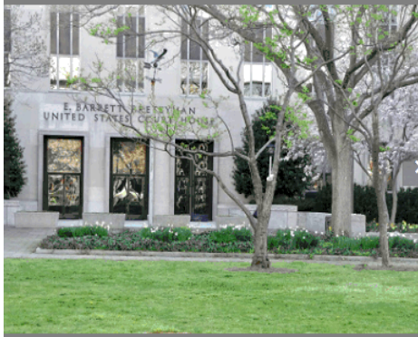
D. C. Circuit Courthouse
